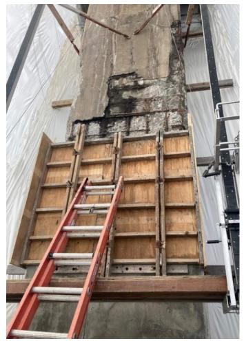
These columns' purpose is to support the structure and all traffic traveling over the bridge. As failure of a column could result in catastrophic failure of the bridge, the construction team needs to take great care and means to assure that during the repair process there are no chances of column failure. During the process of completing the concrete repairs, some of the repairs found were severe enough to require some temporary support of the bridge.
