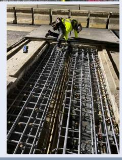
As stated, deck end replacement efforts are completed over the course of 4 to 7 night-time shifts within lane closures. Great efforts are made to complete this work while also allowing unrestricted travel during peak travel hours. To accomplish the task, large steel plates are used to span gaps in the bridge surface and carry vehicular traffic. These plates are designed to carry the heavy traffic loading of tractor trailers, tankers and municipal vehicles that travel the interstate.
