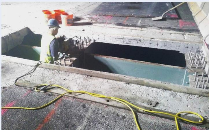
Once drilling and chemical anchoring of horizontal reinforcing is complete, formwork is installed, and the remaining reinforcing is placed.
